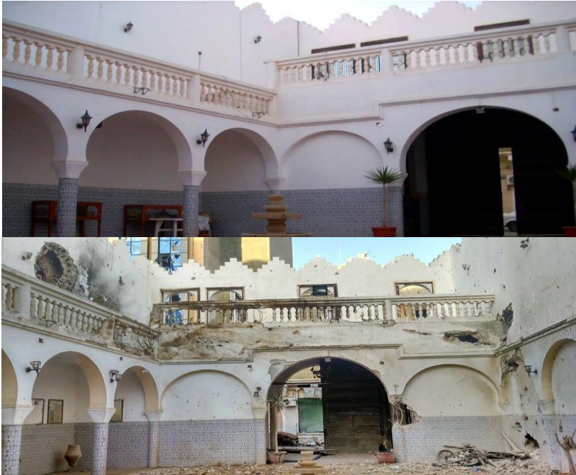
Figure 5: A courtyard in the Saraya before and after a war attack
